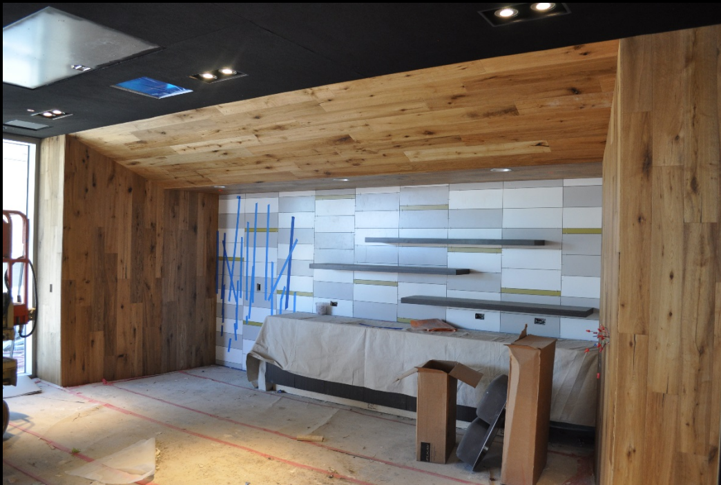
Wood plank and tile backsplash installed at countertop in Club Room
