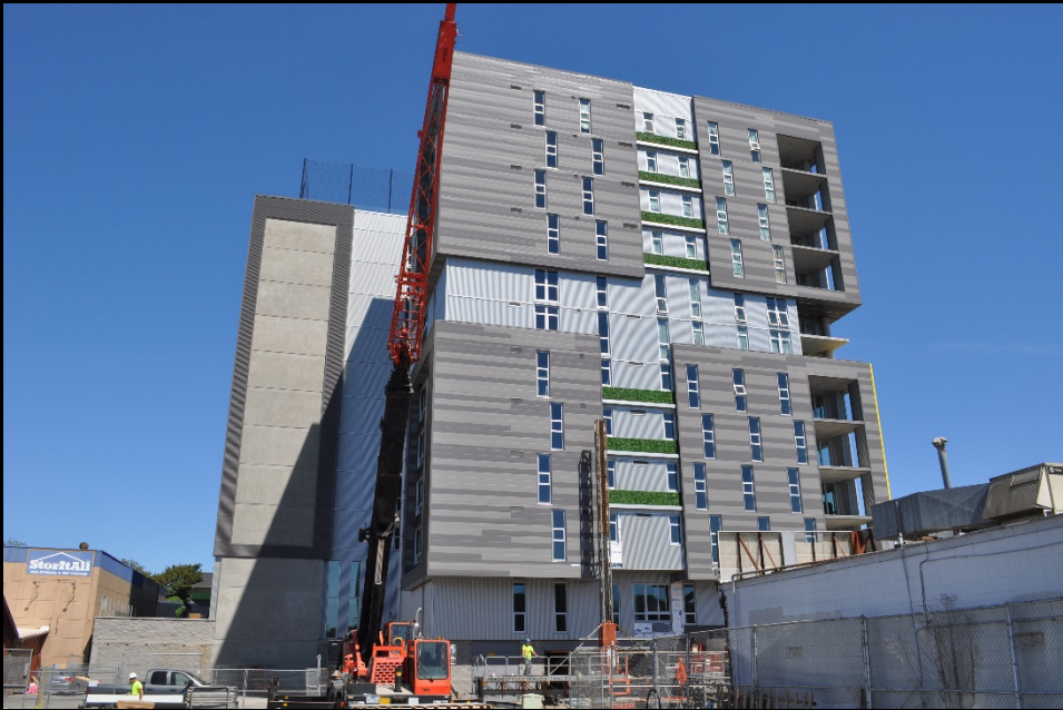
West elevation with ivy installed and Fraco scaffold removed
