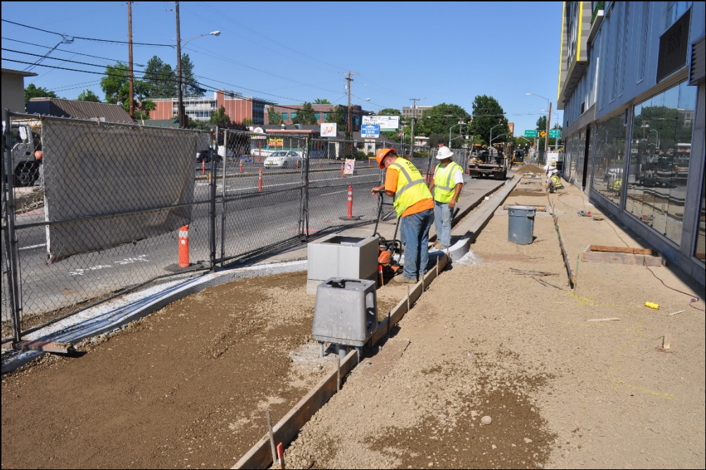
Soil compaction before sidewalk placement at South side
