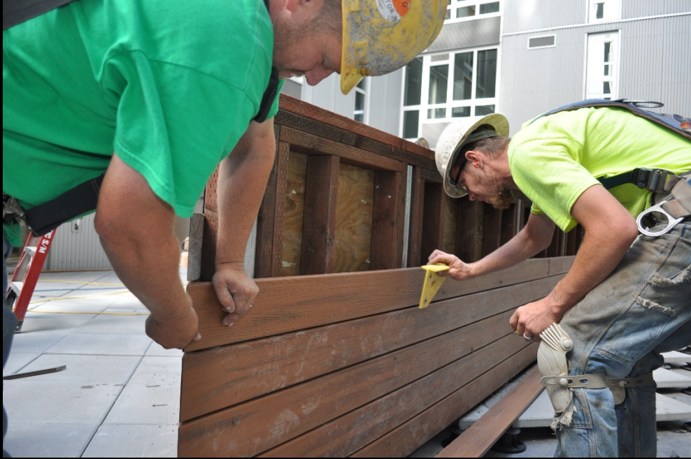
Trex deck installation at Courtyard benches
