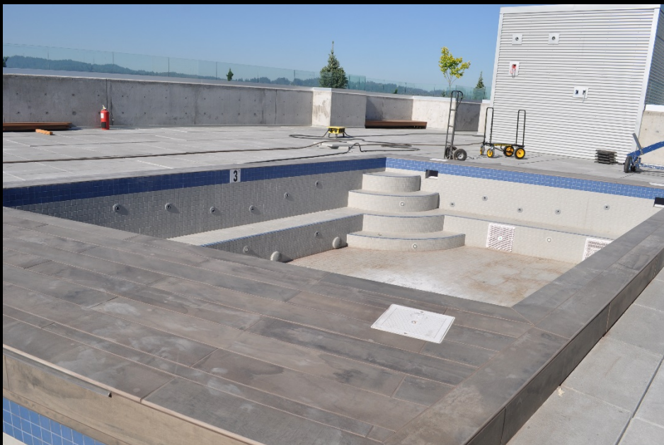
Tile installed around rooftop hot tub
