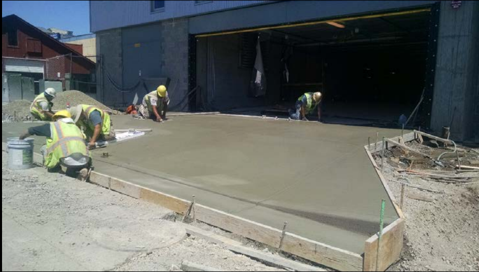
Finishing concrete at driveway approach to Parking Garage
