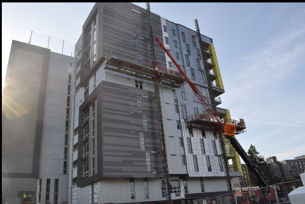
West elevation rigid insulation installed at elevator hoist build back
