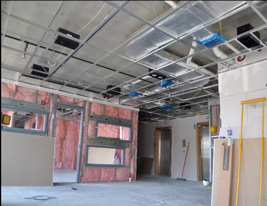
Ceiling rough-in and framing complete and wall insulation installed at level 1 Leasing
