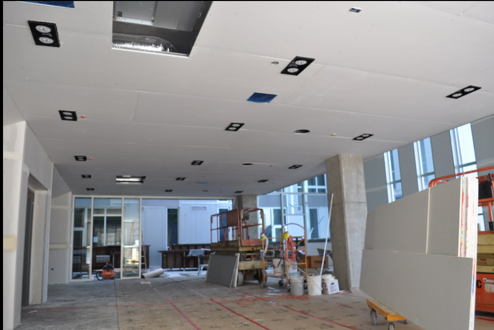
Drywall installed at Club Room ceiling
