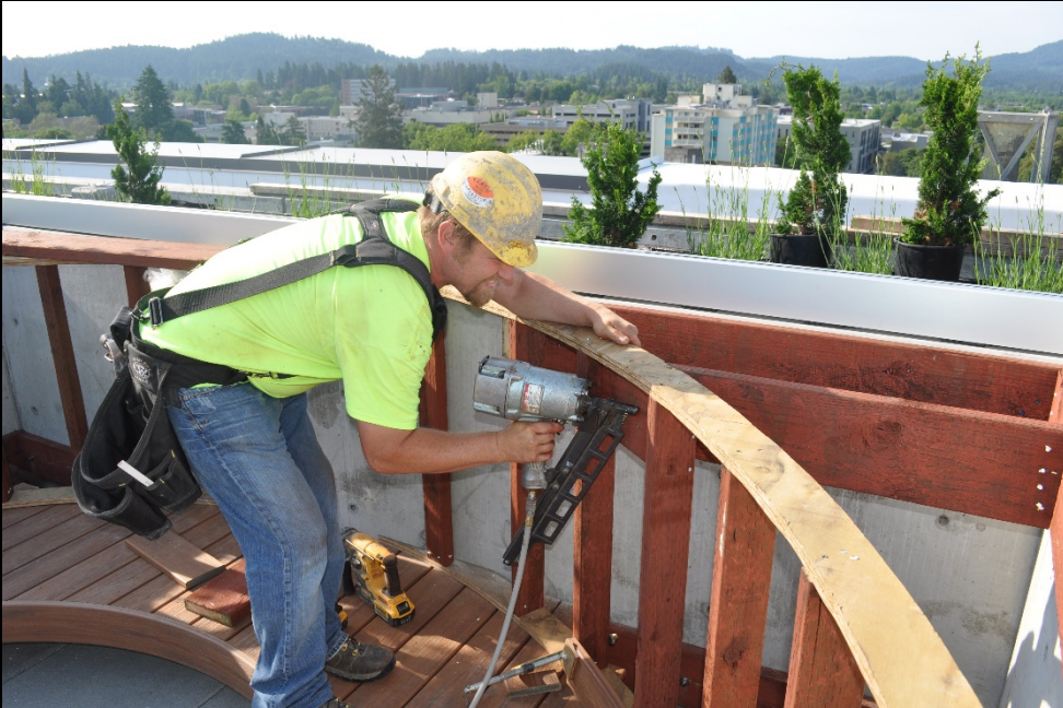
Bench framing at rooftop fire pit
