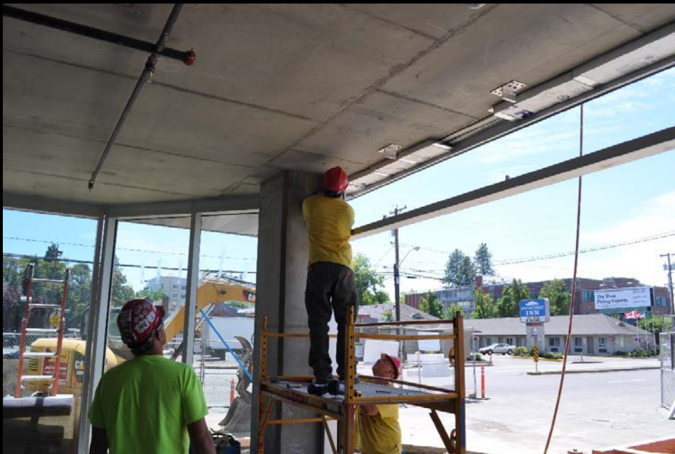
Aluminum storefront install at level 2 Retail space
