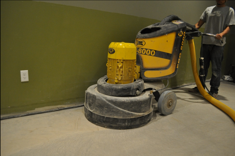
Grinding concrete floors on level 2 before polishing
