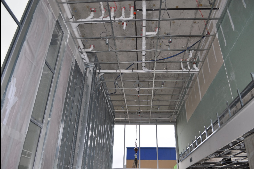
Overhead MEP rough-in and ceiling framing complete at high ceiling in level 2 Club Room
