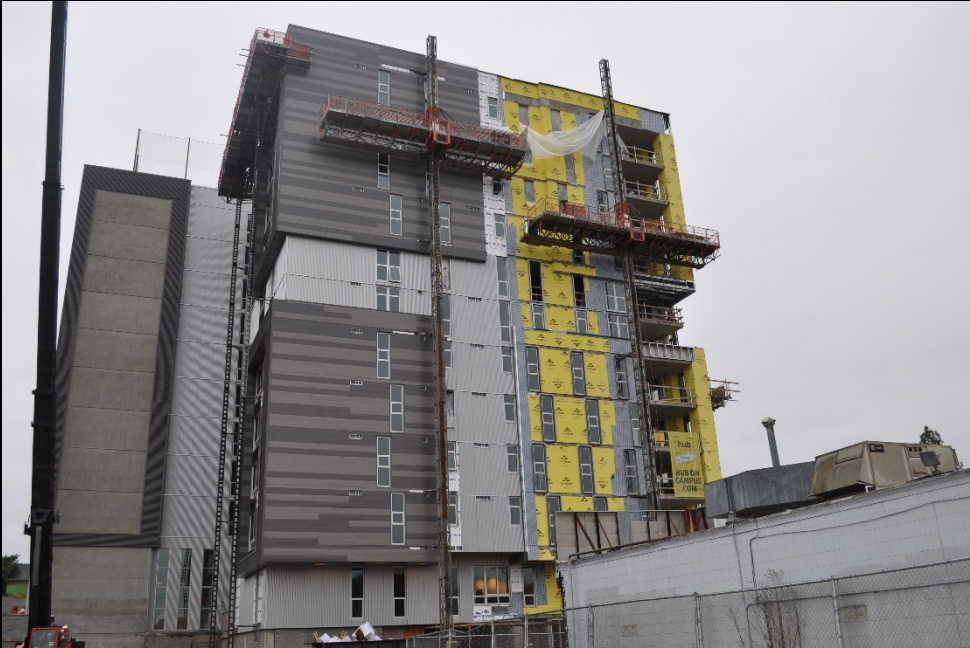
West elevation at elevator hoist build back with windows installed up to level 7
