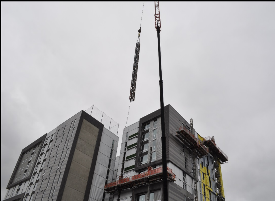
Fraco scaffolding removal at Northwest elevation
