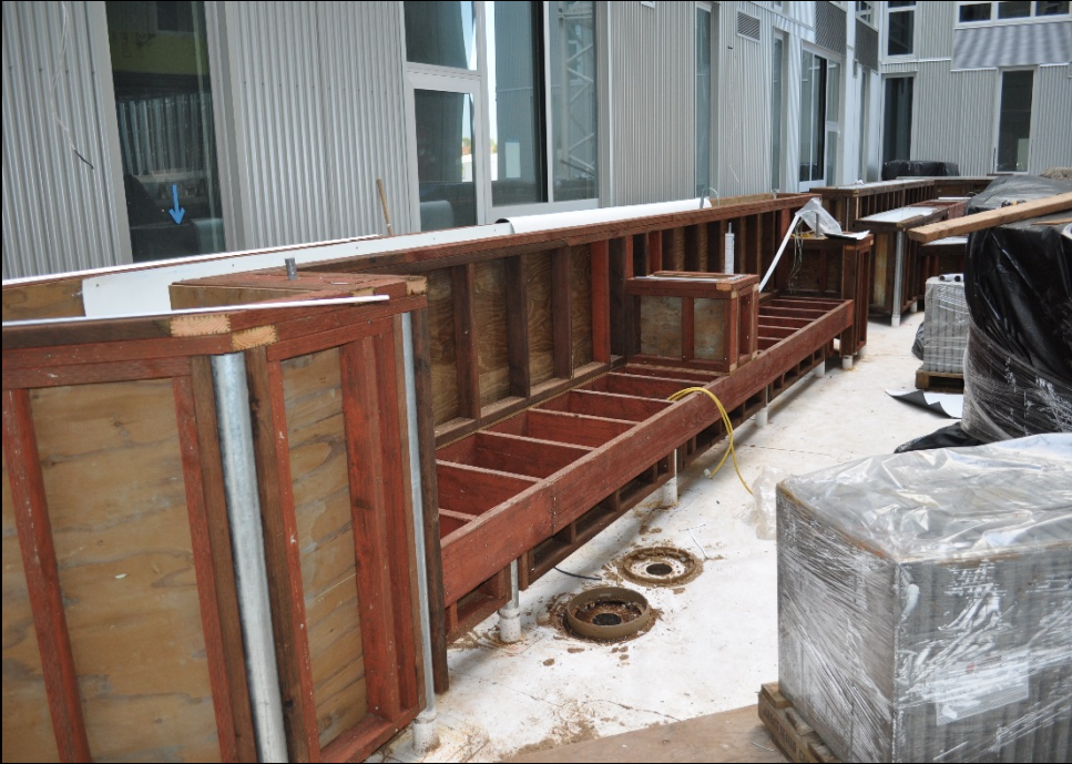
Planter and bench framing at courtyard
