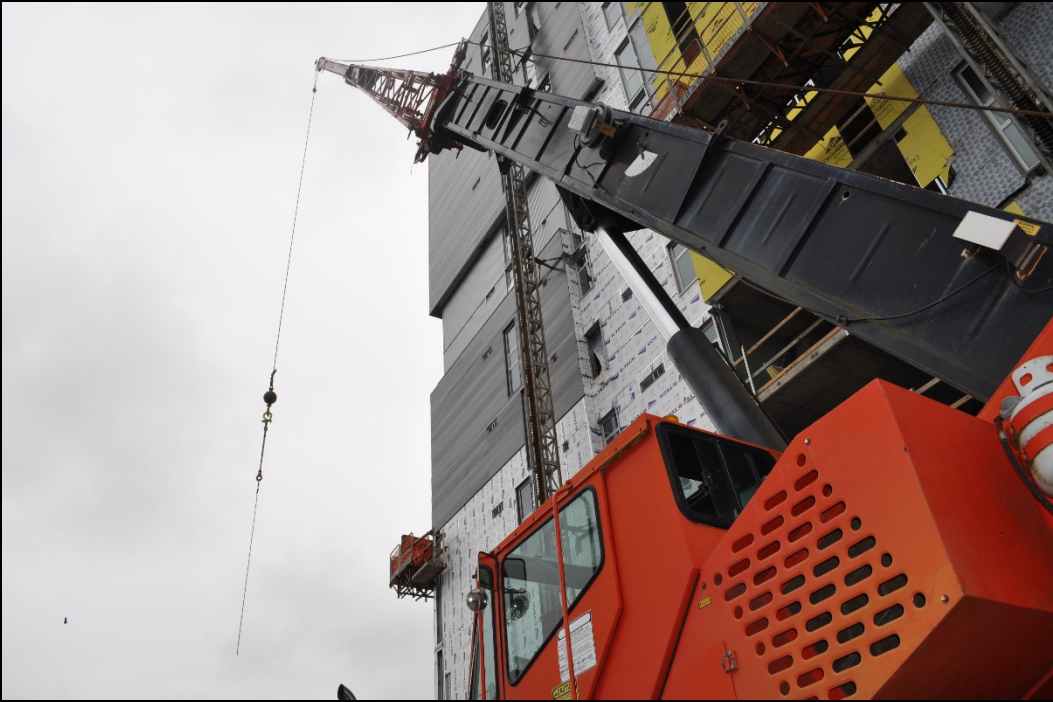
New hydro-crane for material hoisting
