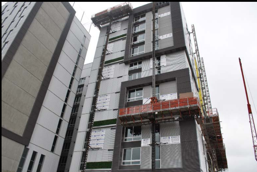
Ivy installed at Northwest elevation
