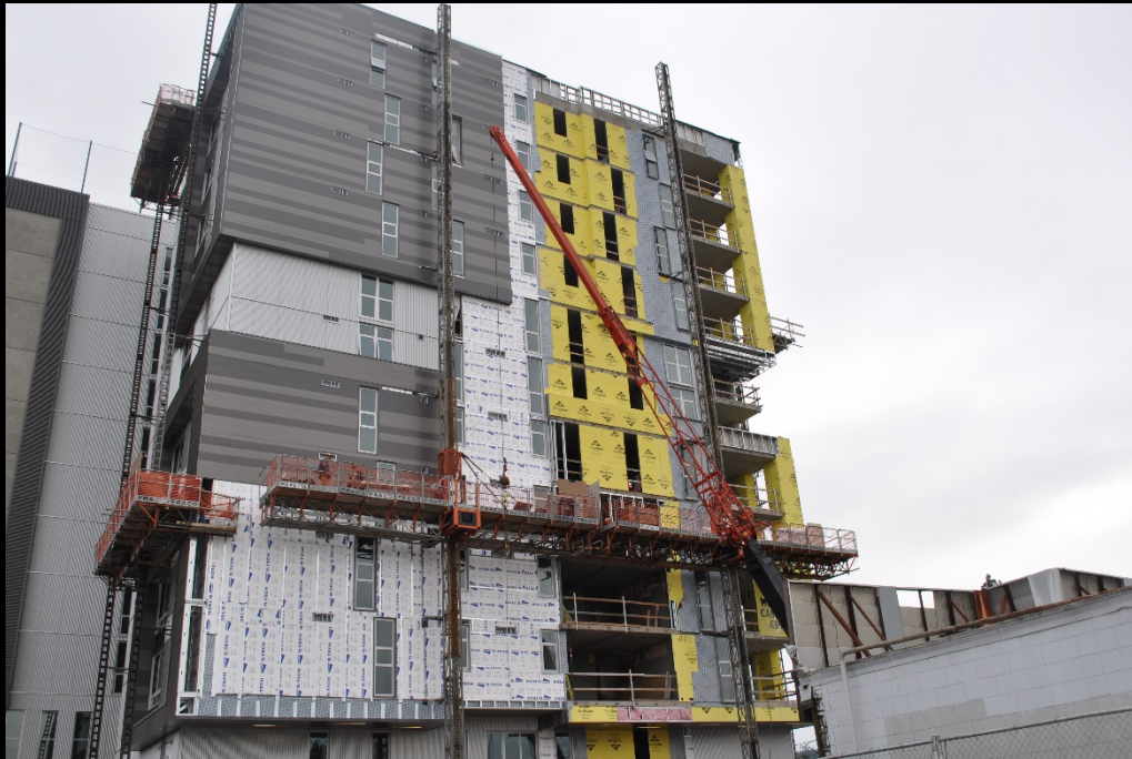
West elevation metal panels and exterior sheathing where elevator hoist was
