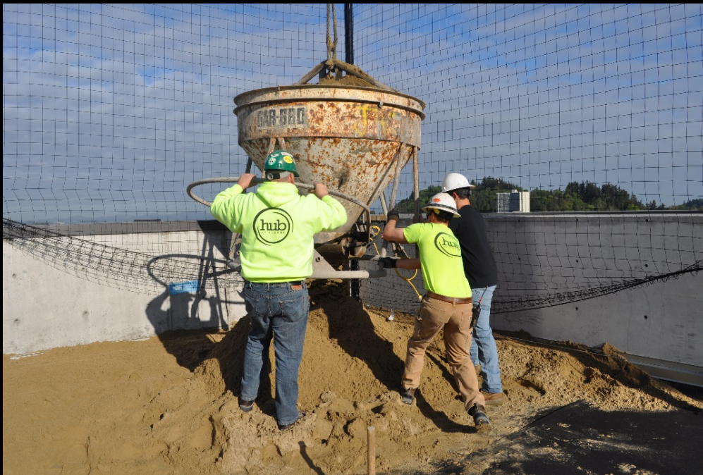
Dumping the sand out of the hopper on to the court
