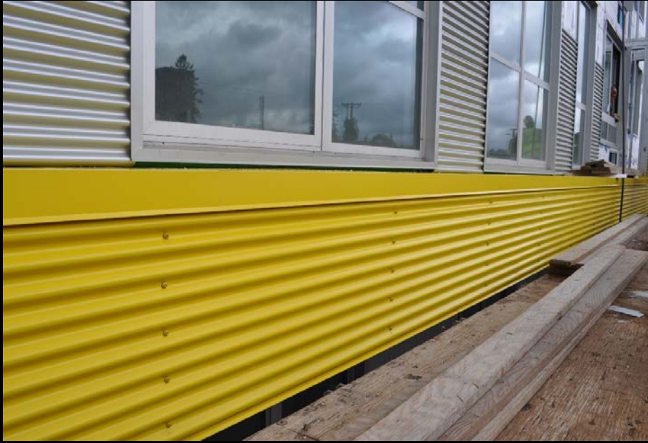
Corrugated metal panel at yellow bump out on South elevation
