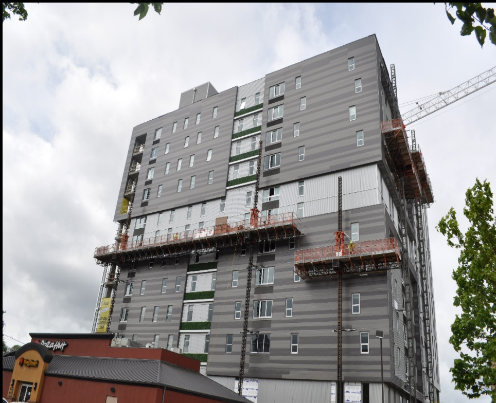
Ivy installed at East elevation. Fraco scaffolding being removed.
