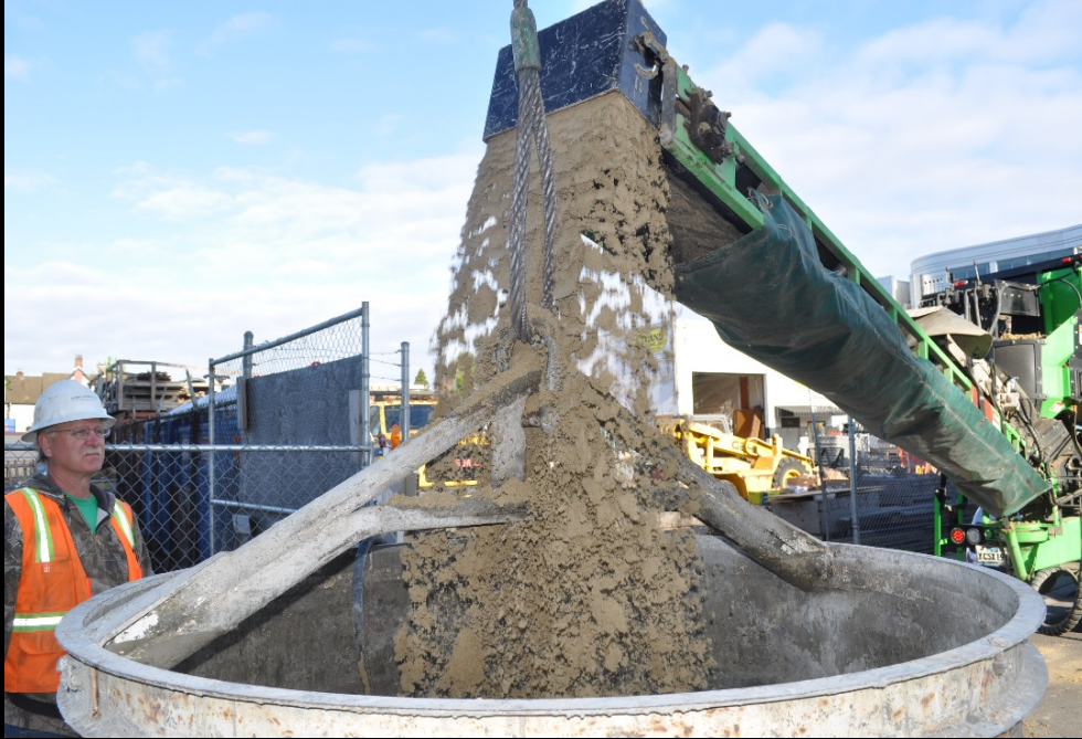
Dropping the sand into the hopper for the rooftop volleyball court
