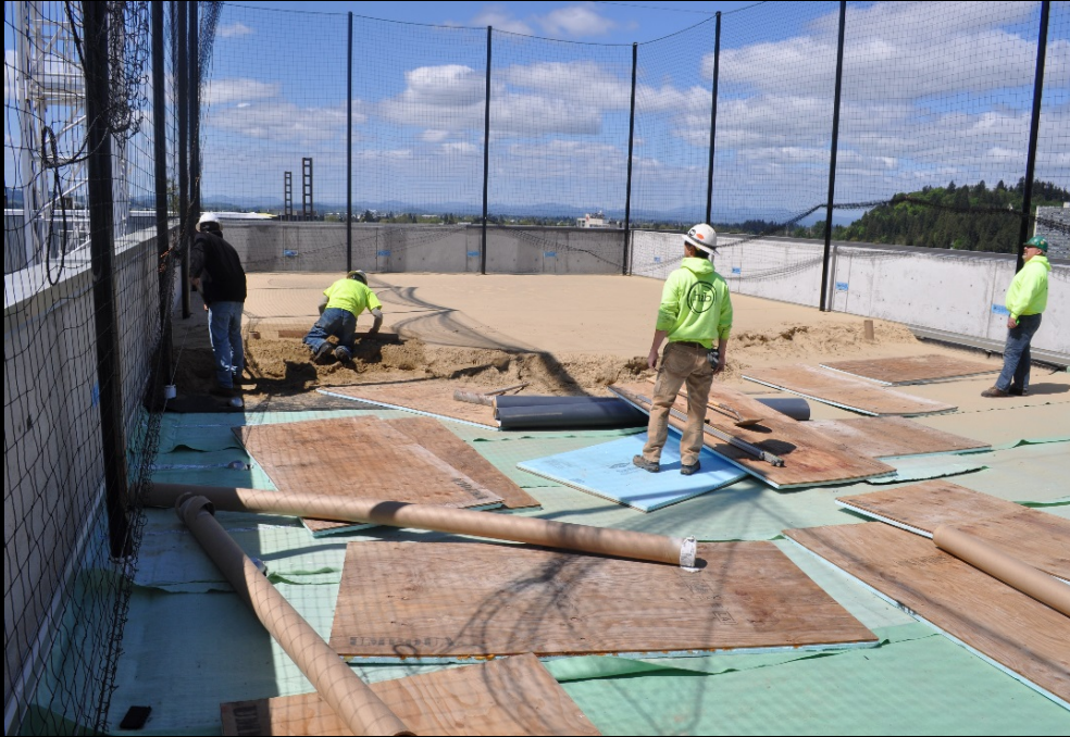
Leveling the sand by hand
