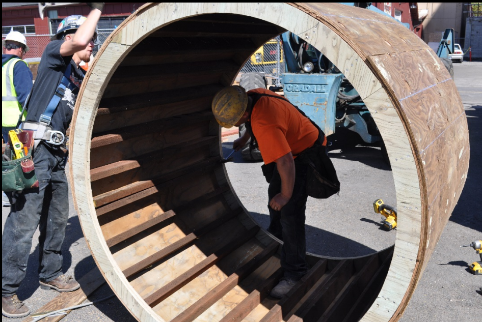
Building radius form for tree planter at courtyard
