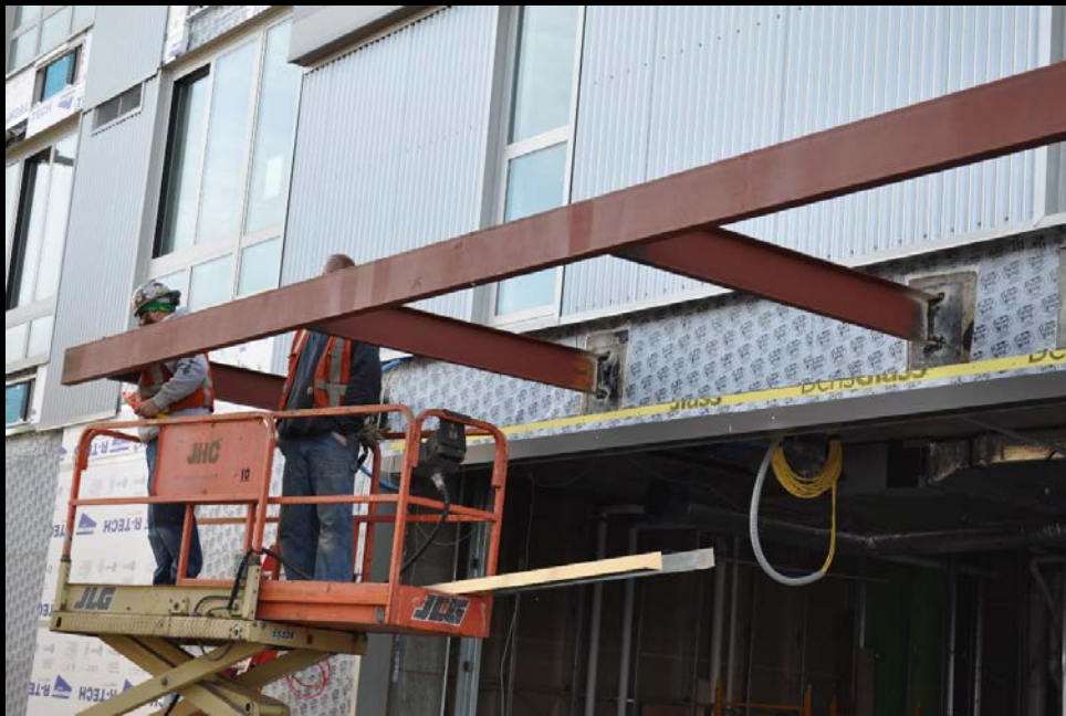
Installing steel canopy at outside club room on 2 nd floor
