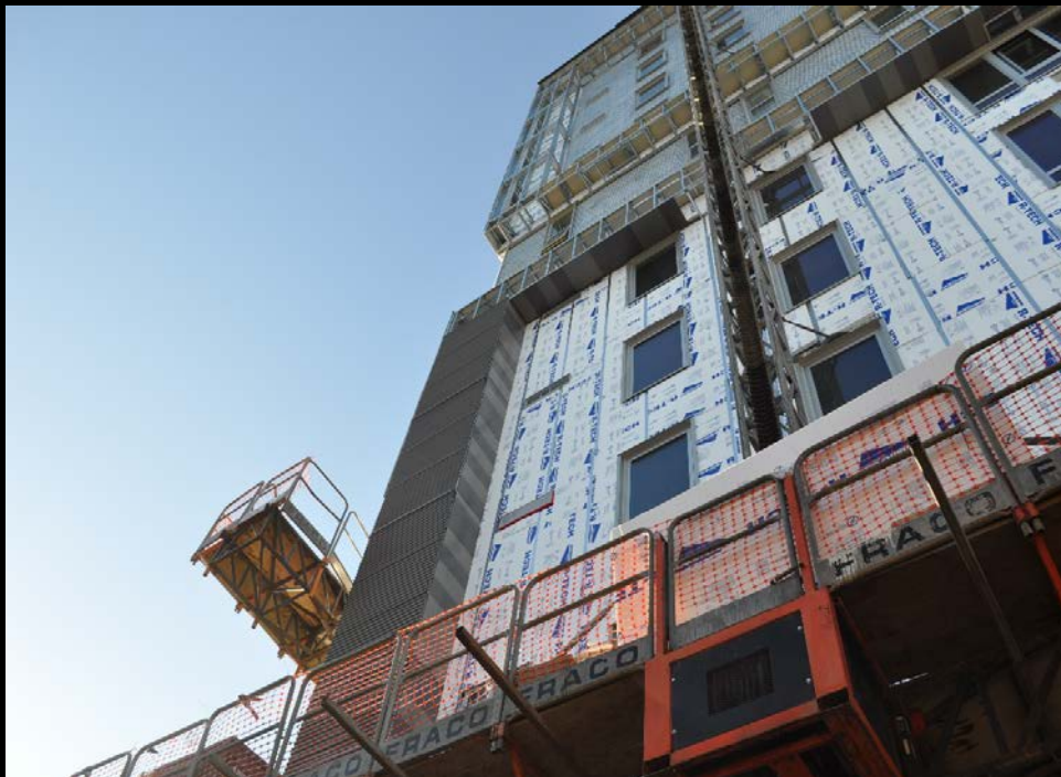
Corrugated metal panels installed at bump out on North elevation
