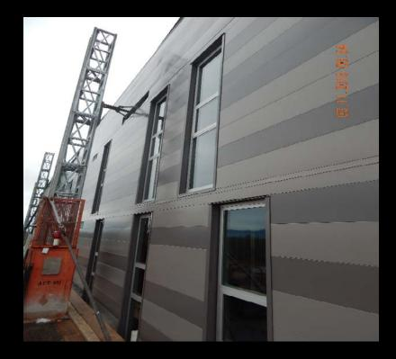
Linear metal panels at North elevation
