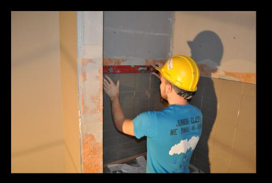
Ceramic wall tile installation 2<sup>nd</sup> floor bathroom
