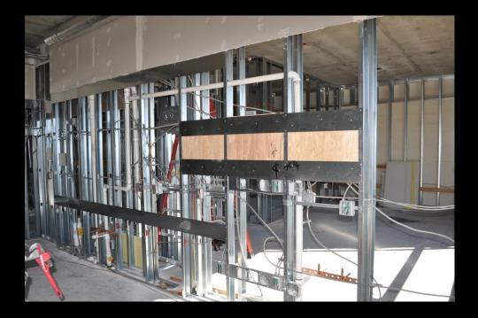
Level 2 kitchen/living room wall backing for casework and TV installed.
