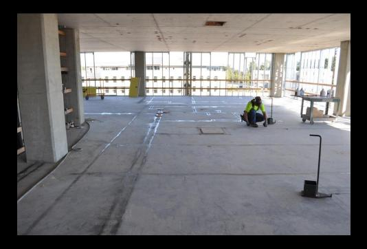
Level 5 south east corner view to the north interior wall layout in progress.
