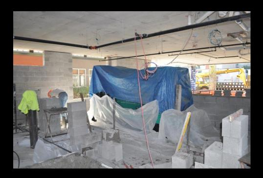
Electrical back-up generator in place CMU underway to complete the enclosure.
