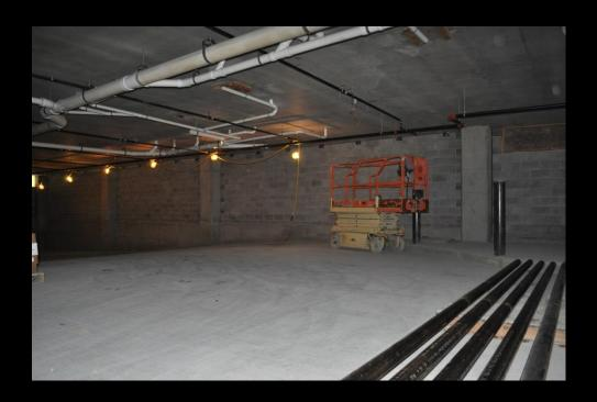
Level 1 parking garage looking north east down ramp to basement, CMU walls complete.
