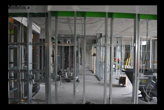
Level 4 north side of the building looking west, prerock complete at ceilings and electrical rough in underway.
