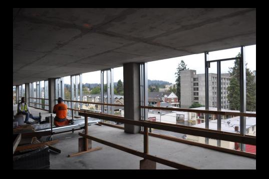
Level 5 south exterior wall framing complete.
