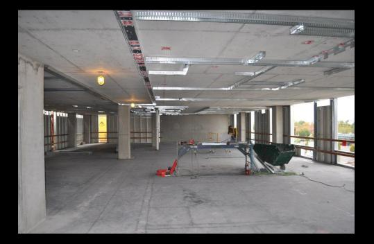
Level 5 north side of building view to the west, interior framing underway with ceiling track installed ready for wall studs.
