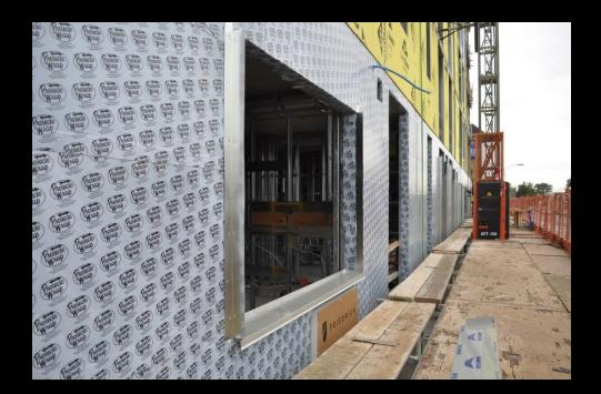
Window flashing and weather barrier level 2 south elevation
