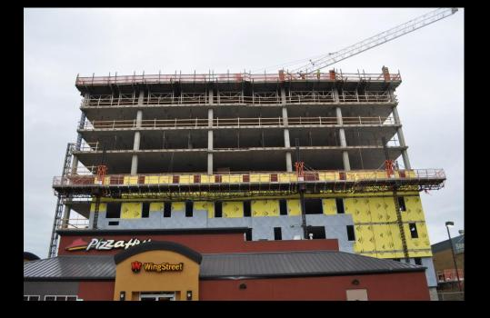
East elevation, exterior Dens-glass to level 5, weather barrier in progress
