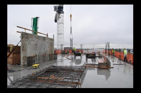
Level 12 north east corner looking west. Installing column reinforcement.
