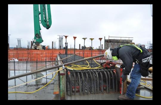
level 12 pool support beam formwork and reinforcement
