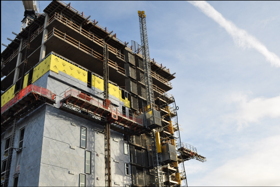
Two-cab elevator extended to upper levels
