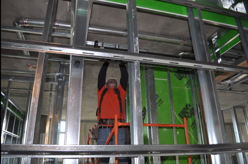
Interior wall framing level 7
