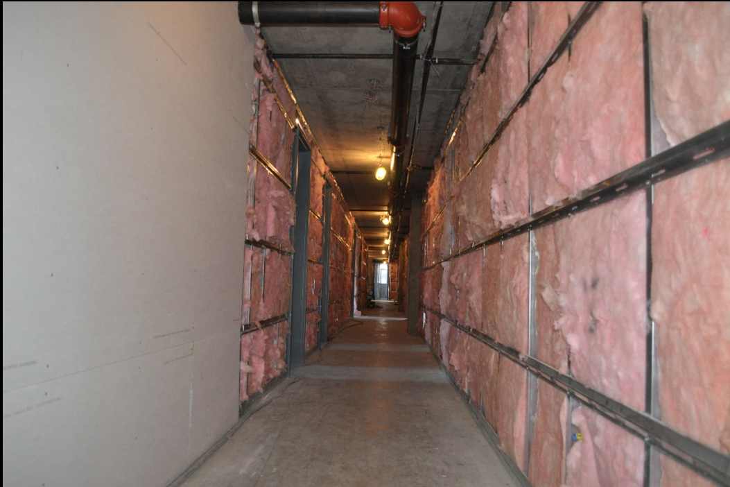
Wall insulation on level 3
