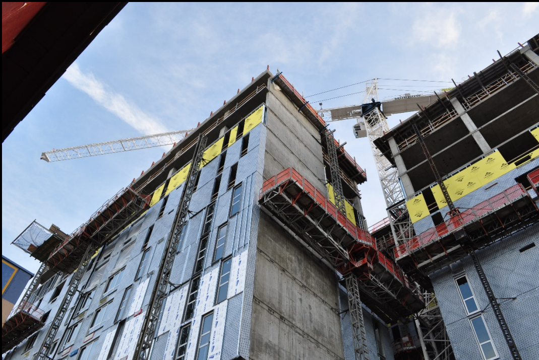
Rigid insulation at North elevation
